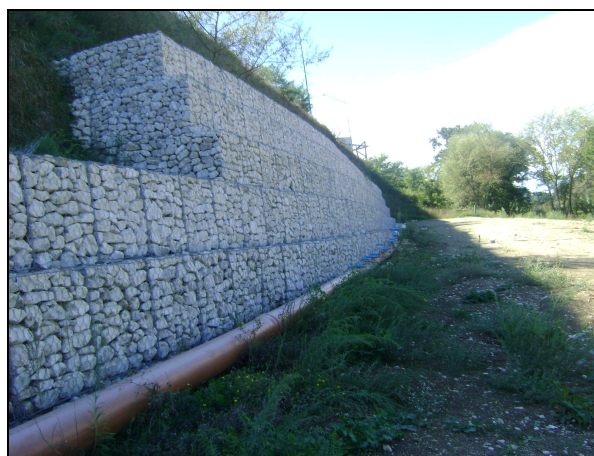
Fig. 2 – Provisional safety measures intervention: installation of metal gabions.
