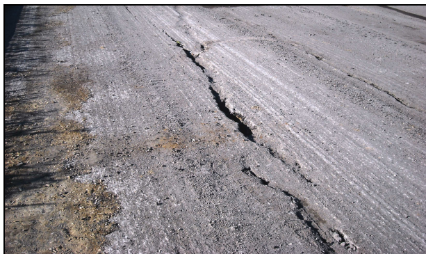
Fig. 1 – Damage on the road as a result of the collapse occurred.
