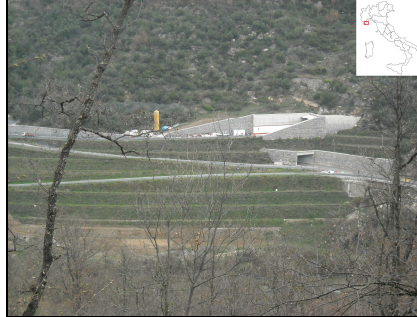
Fig.2.2.1 - Overview, from the opposite slope, of the road interchange
