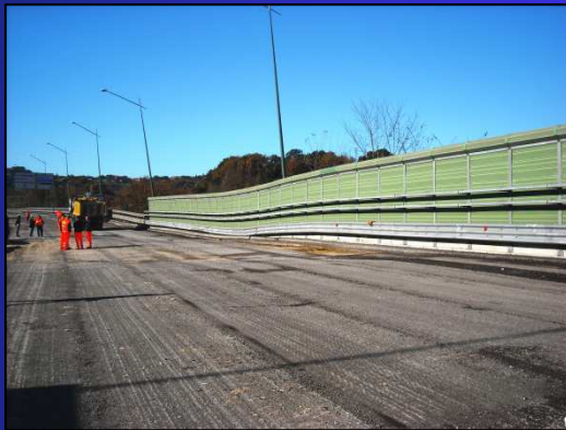
Overview of the deformed roadway
